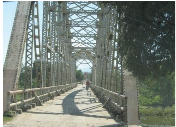
The Jutiapa bridge in more recent years
