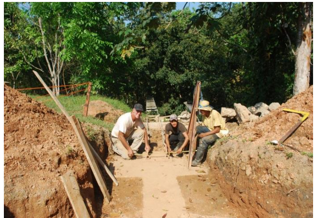
bridge renewal in process
